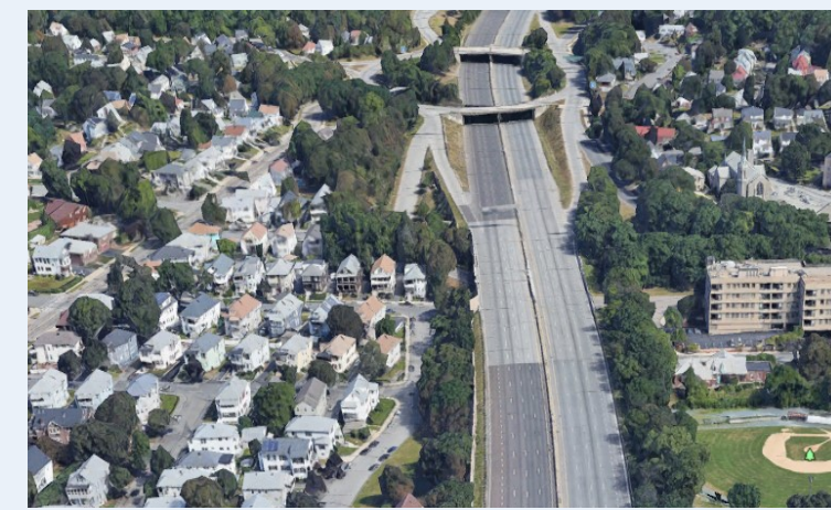
Route I-93 in Medford borders homes and play areas. Regional highways that were inserted into older urban neighborhoods are a source of noise exposure in Massachusetts.
