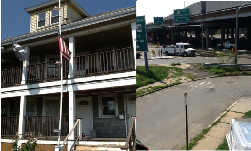
Figures 38 (a) and (b) – note: highway noise barrier at top of photo on right, above sign
